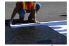
Fig. 6 Position PreMark® material according to diagram provided.
