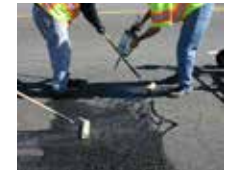
Fig. 5 Squeeze out sealer and spread with roller.
