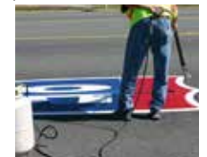
Fig. 7 Heat PreMark material
