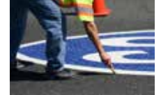
Fig. 2 Position marking to draw outline of application area
