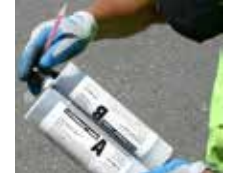
Fig. 4 Prepare sealer cartridges for use in sealer gun.
