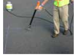
Fig. 1 Prepare area by removing debris with blower then remove moisture with heat torch
