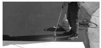
Heat HotTape™ with a propane heat torch such as the Magnum Heat Torch.
