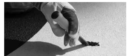
Chisel test to ensure proper bond.
