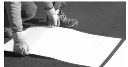
Clean the surface to remove any debris. Preheat the pavement surface to a minimum of 300° F.
