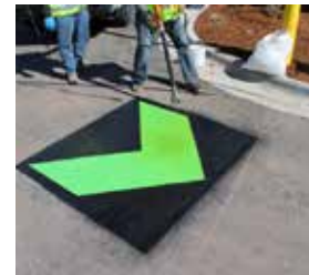
Heat with propane heat torch according to instructions
